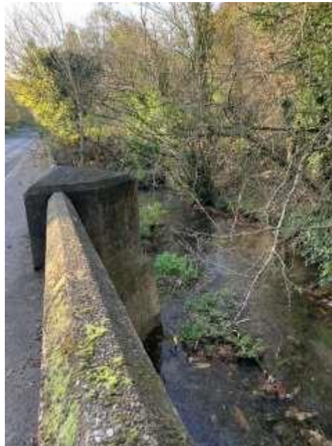
Semington Brook Bridge
