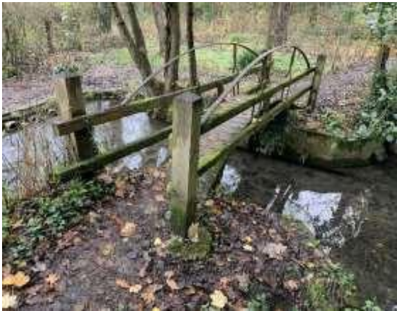
Bridge at Home Farm
