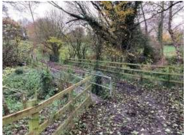
Bridge at Whites Mill
