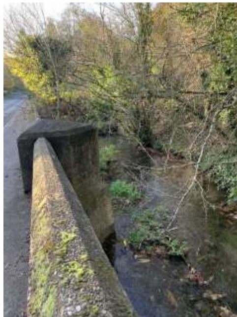
Semington Brook Bridge
