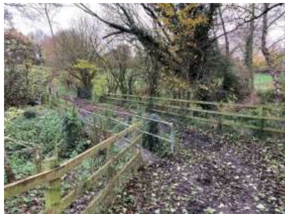
Bridge at Whites Mill
