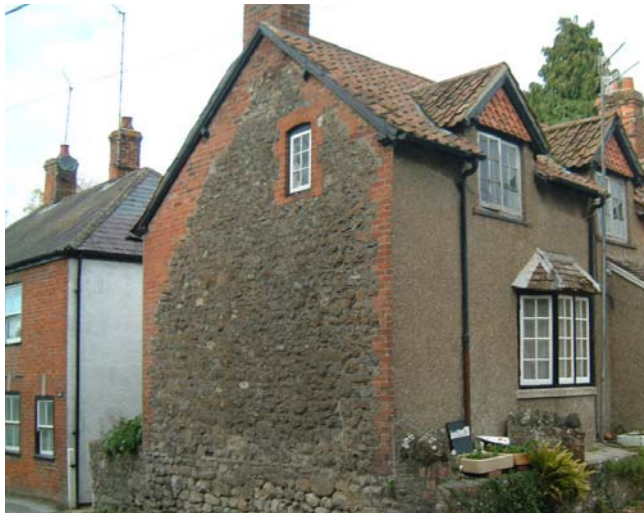
A cottage gable originally constructed in Greensand stone for a steep pitched roof, probably thatched, was raised in brick to improve the interior and tiled.
