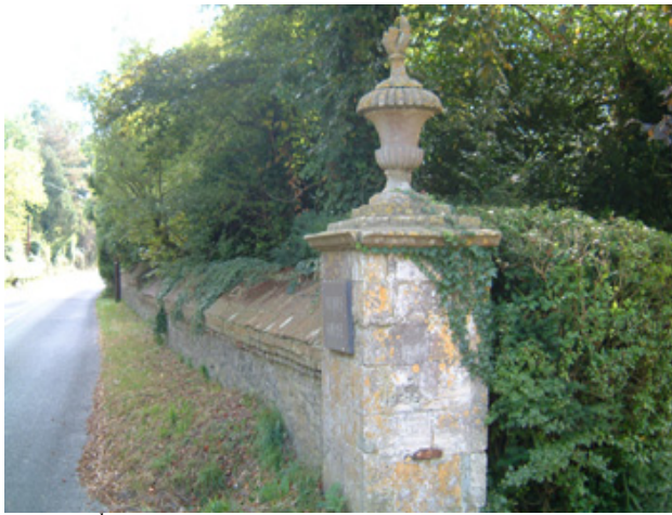
The 18 th century Greensand stone wall with brick coping and a limestone gate pier to Hunts House.
