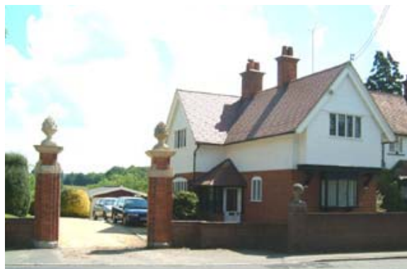
A'Beckett's Lodge was built with the house in 1904. The gatepiers and finials are recent.
