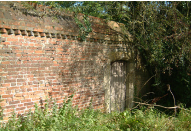
The 16 th century garden wall of West Lavington Manor. Brick with a deep coping and a cogged
