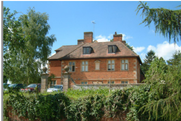
The 17 th century east wing of A'Beckett's was restored and extended into a mansion in 1904
