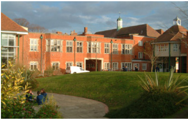
Dauntsey's School. The Quadrangle garden and extension buildings of 1936 and 1997
