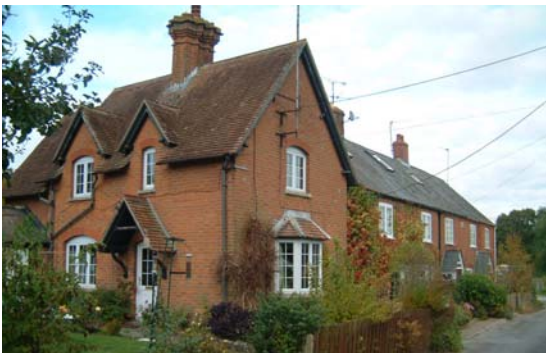
Mid 19 th century Cottages Russell Mill Lane Littleton Panell
