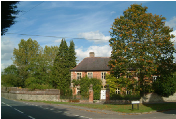
The roadside wall on the A360 and Dial House facing a small green at the junction with Rutts Lane
