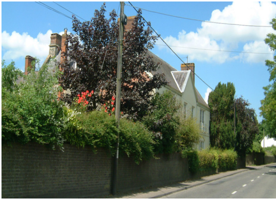
Littleton House has an elegant early 19th century front but is of 17 th century origin.
